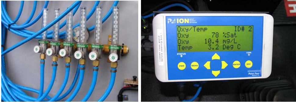
ABOVE: The control station located at the rear of the trailer allows drivers to control the flow the oxygen levels through the six tanks from their cab, ensuring there is plenty of oxygen for the salmon during transit between the sea farms and hatcheries.
