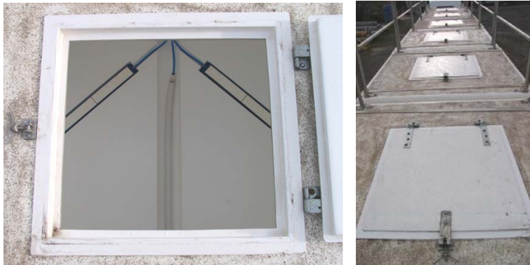
ABOVE: A view from above of the tanks.
